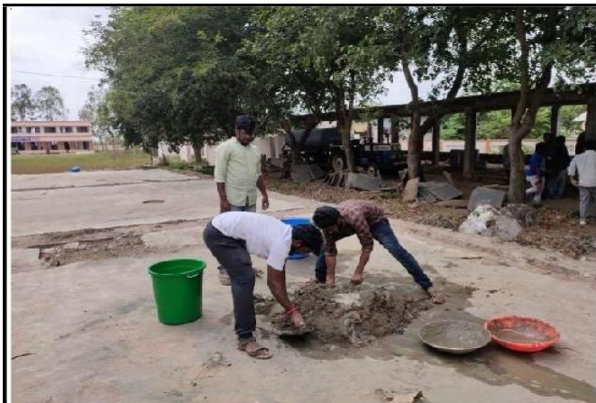
Students mix up sand and cement them in a correct ratio for the wall.
