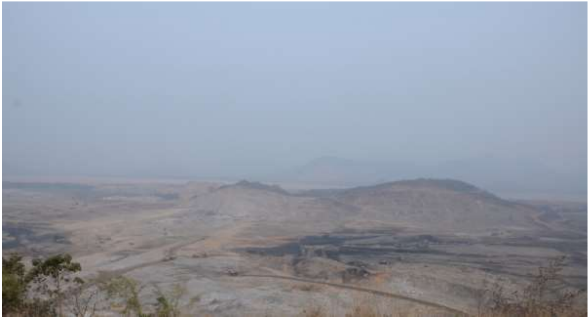
FIG: 6. CONSTRUCTION SITE VIEW OF POLAVARAM PROJECT.
