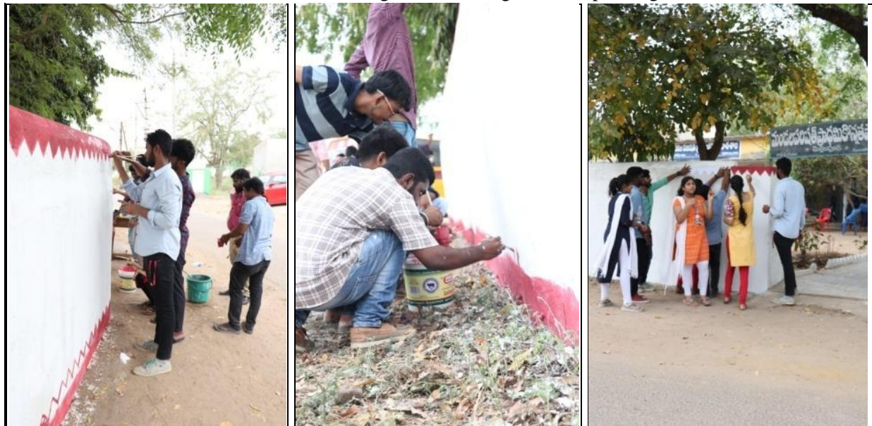
School building wall Cleaning and wall painting
