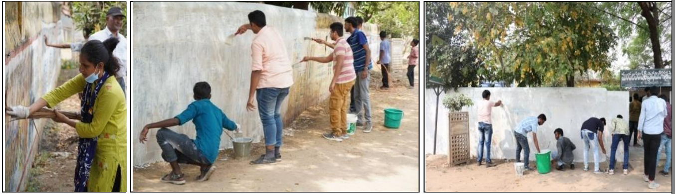
School building wall Cleaning and wall painting
