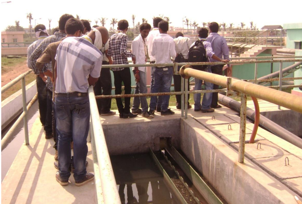
Students observing up flow anaerobic sludge blanket tank
