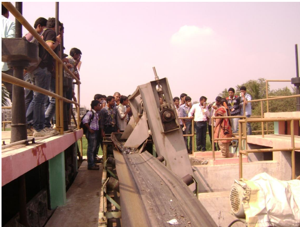
Engineers of waste water treatment plant explaining screening and automatic cleaning
