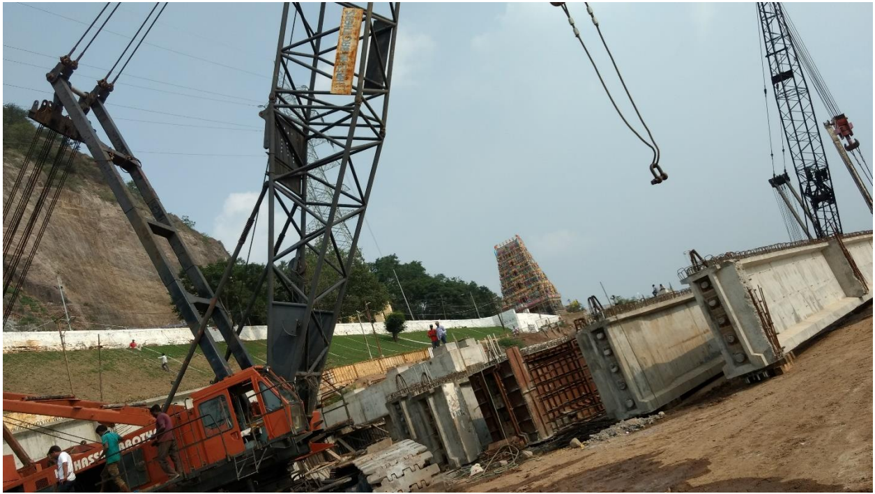
ERECTION OF PRE-CAST GUDDERS
