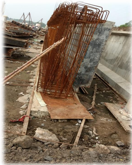
REINFORCEMENT FOR PILES AND PRE-CAST GUDDERS
