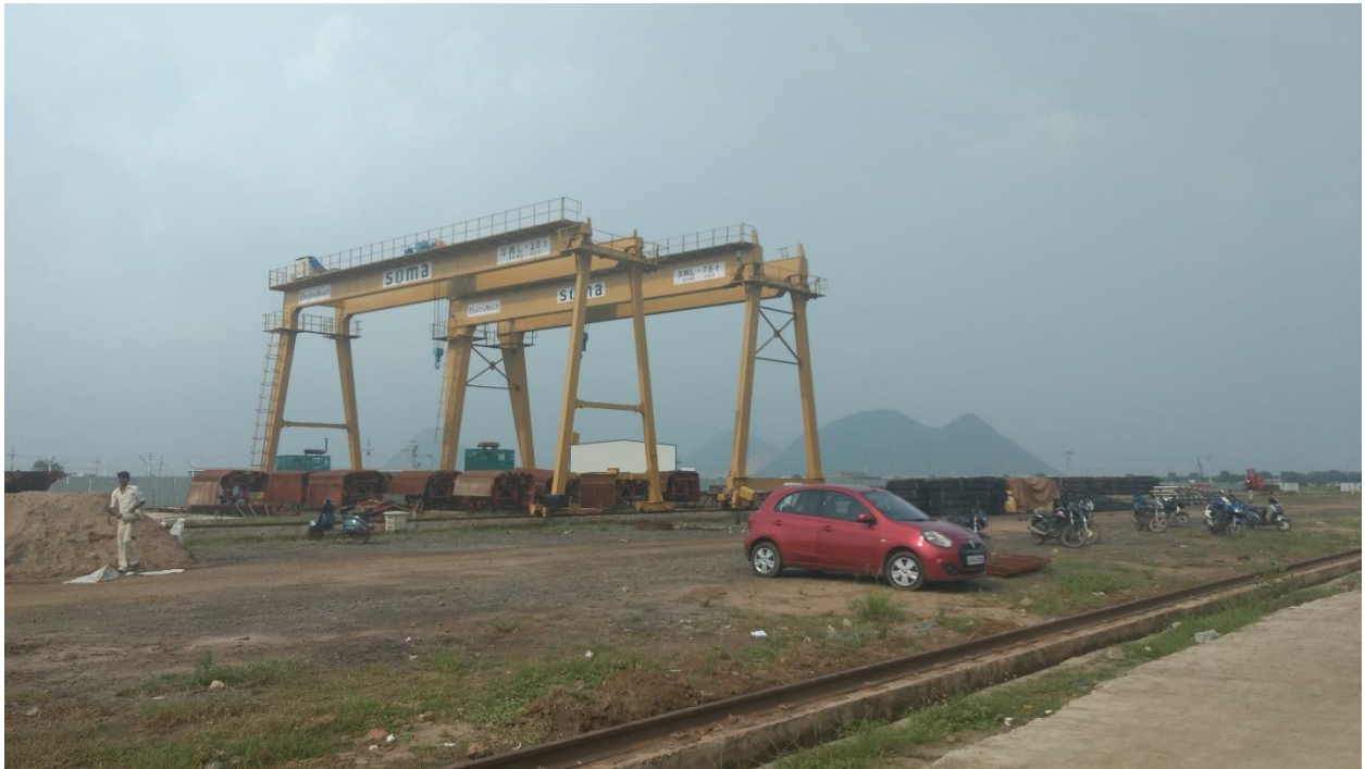
HIGH CAPACITY CRANES ON THE PRE-CAST PLANT
