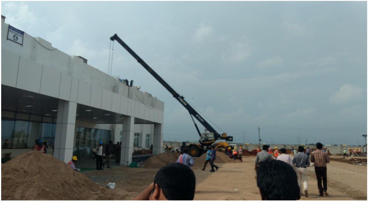
ERECTION OF PRECAST BEAMS USING CRANES
