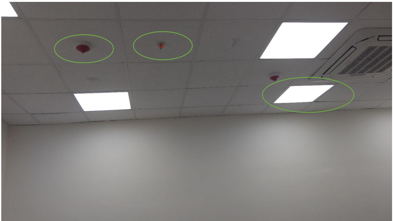
FIRE SAFTY SYSTEM AND LED LIGHTS INSIDE THE BUILDING
