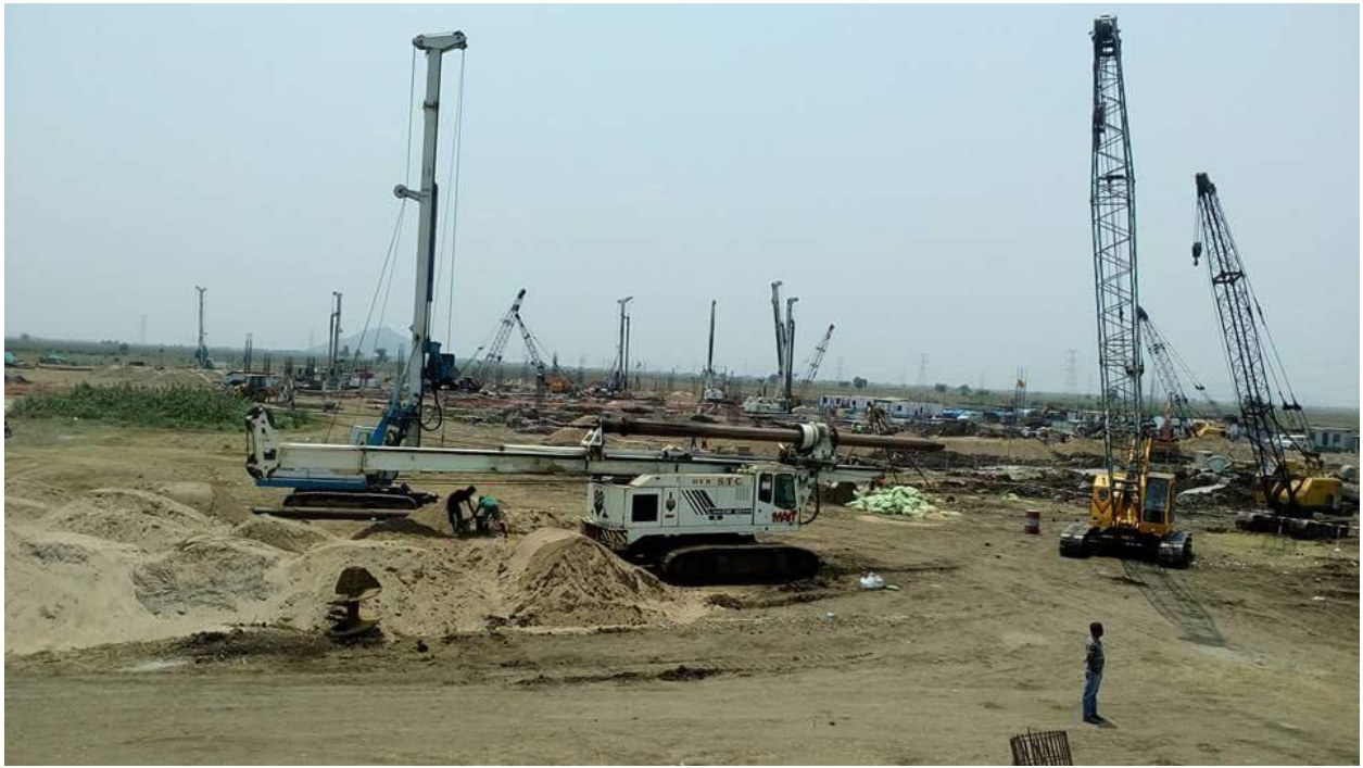
HUGE NUMBER OF PILING WORK FOR FOUNDATION WORK
