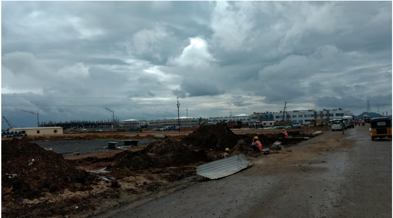
A VIEW OF VELAGAPUDI SECRETARIAT CONSTRUCTION
