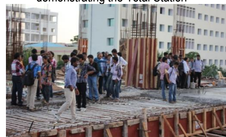
Field visit to Library Building for demo on Radiant Cooling Technology
