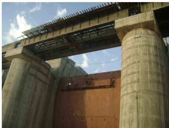
radial gates and bridg deck
