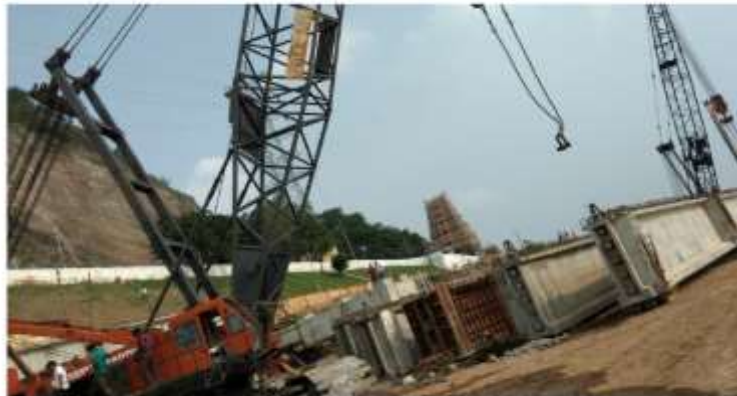
ERECTION OF PRE-CAST GUDDERS
