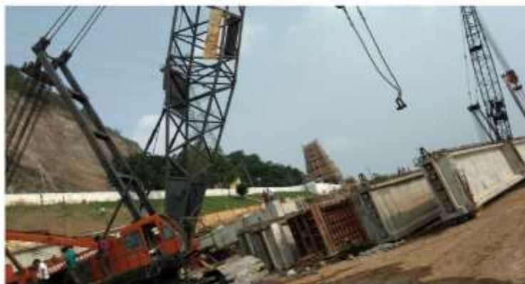
ERECTION OF PRE-CAST GUDDERS
